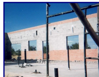
Walls going up
